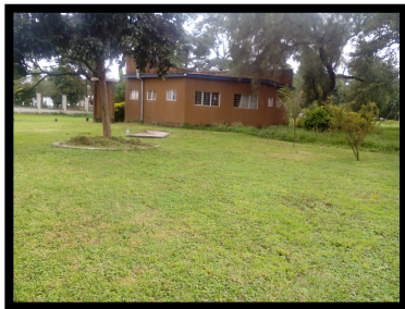
Toilet at Arusha Peace Park
